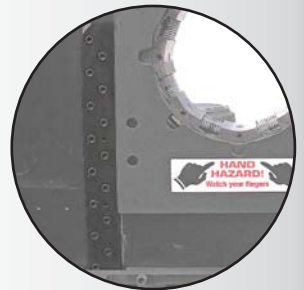
Inspection & Cleaning of Side Guide Plates
